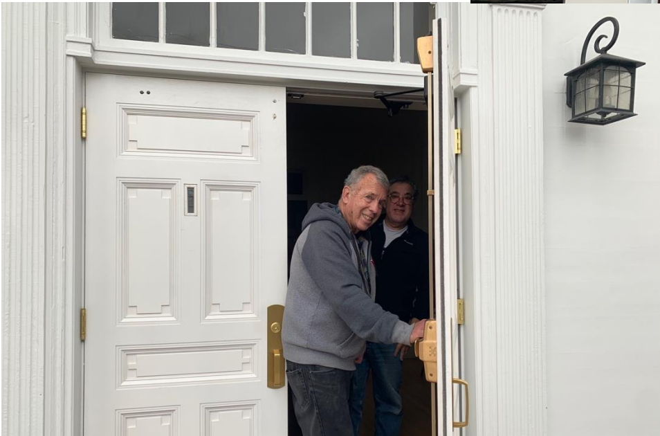
November 16, 2022 - Clif Holbrook (Member & House and Grounds) and Peter Bianco (Maintenance Officer) inspect the new doors
