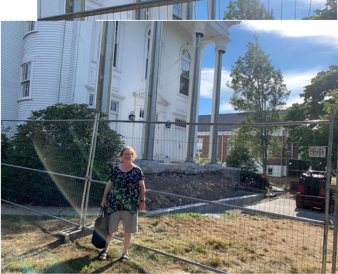
Liz Mercer in front of FBC Needham – front porch restoration 2022
