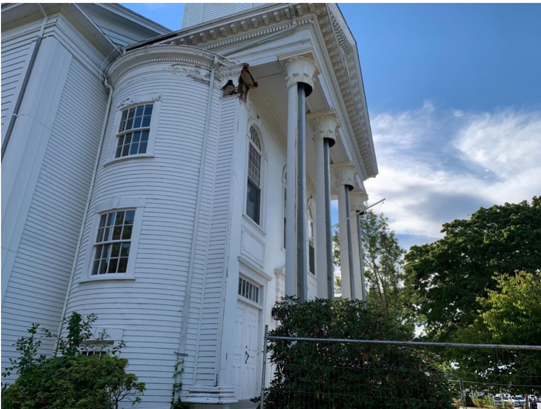
Columns in waiting for the anticipated new porch and stairs
